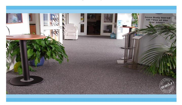
Eradur® Dekor EF can be likened to a stone mat, where a natural stone or polished marble-gravel in size 3-4 mm or 4-8 mm are glued together to an open coating. The natural stone gives the floor a very attractive appearance, with a great variety of possibilities regarding color and pattern. The binder is a solvent-free, clear epoxy.
