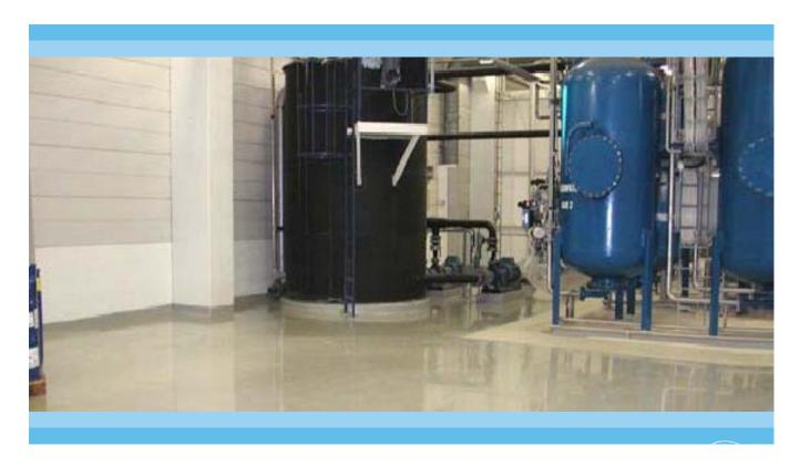
Eradur® PU750 Massiv is a smooth and hard polyurethane coating with good abrasion resistance.
