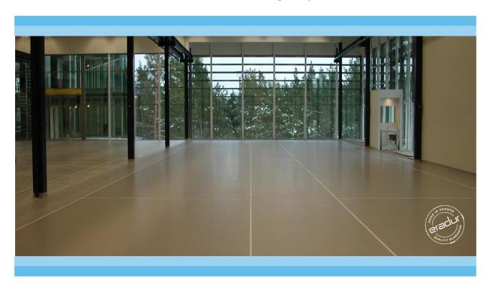
Eradur® Terrazzo is a seamless terrazzo-floor made of solvent-free epoxy with marble, granite, flint or stained glass. It is possible to add a variety of other decorative components that allow for a unique design.
