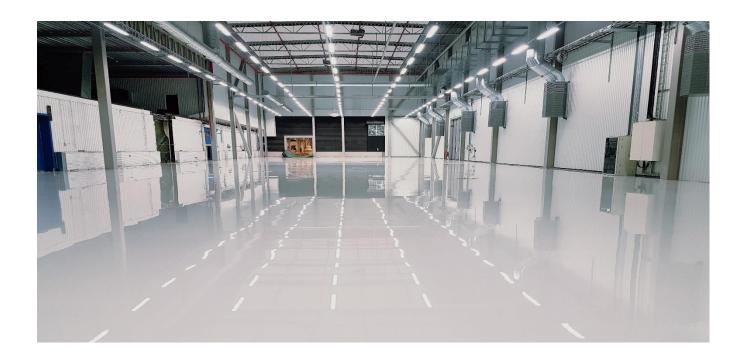
Eradur® ESD Massiv SL is the anti-static version of Eradur® Massiv SL with otherwise equal properties.
